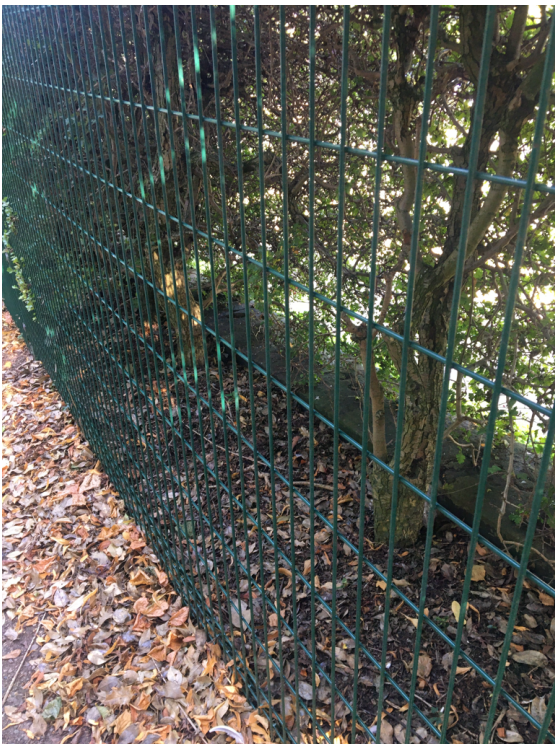
Weldmesh fence on garden-side of existing hawthorn hedge
